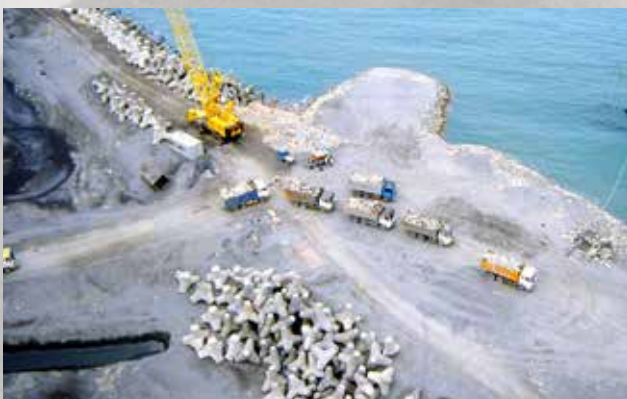
| Border dike construction
